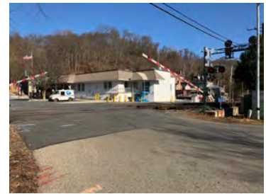
Figure 16 Railroad crossing gates at Center St./Rowland Dr.
