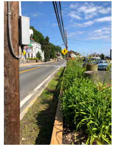
Figure 49 Gap in sidewalk between Marina Park entrance and downtown Port Deposit across from Town Hall.
