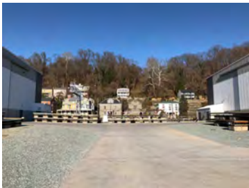
Figure 9 Existing marine commercial
