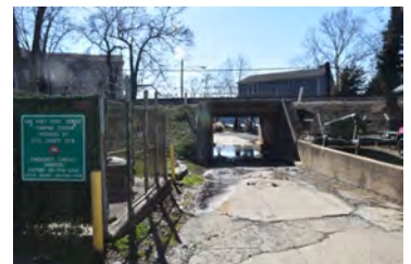
Figure 18 Vannort Dr. railroad underpass
