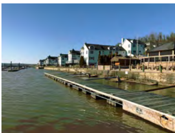
Figure 10 Existing waterfront condominiums and restaurants within the marine commercial zone
