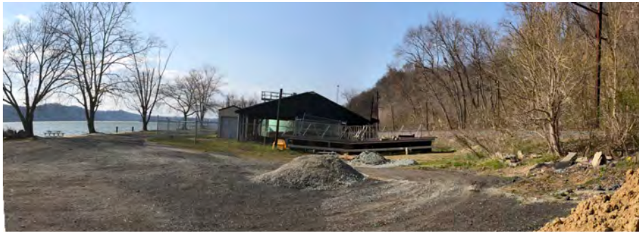
Figure 58 Existing sewage treatment facility to be relocated out of floodprone area
