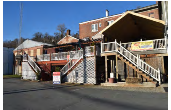
Figure 39 Existing upper floor dining facing the waterfront
