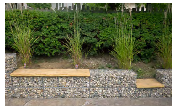
Figure 72 Examples of seat walls in floodprone areas
